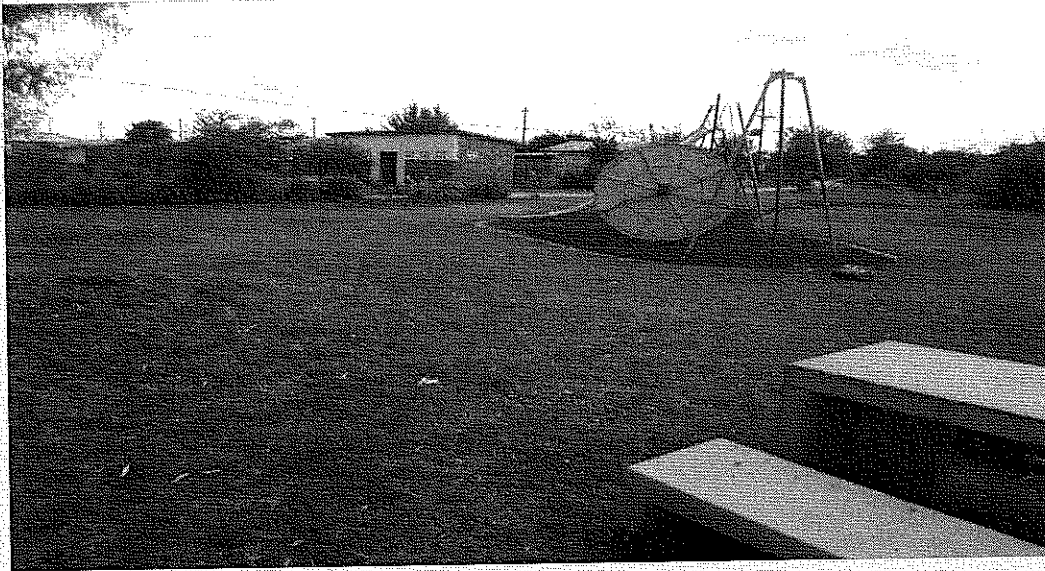
PICTURE: 10 ABLUTION FACILITIES AT PIENAARSRIVIER PARK
