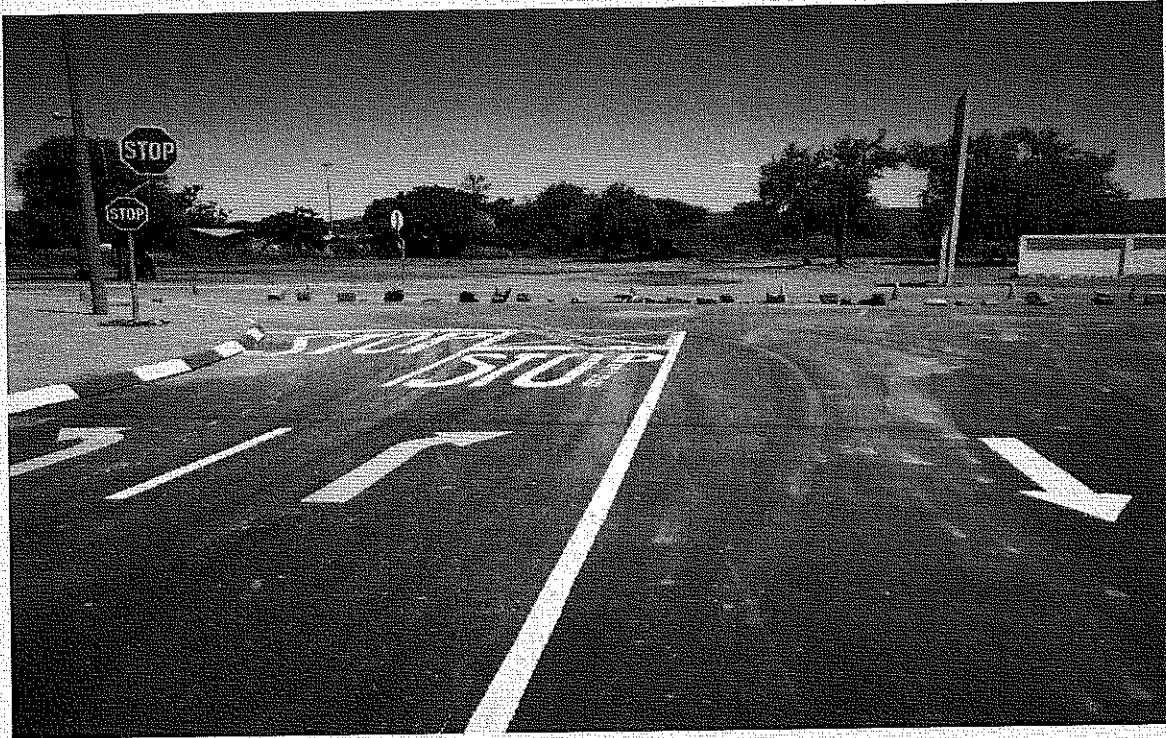
Upgraded road at Mile street
